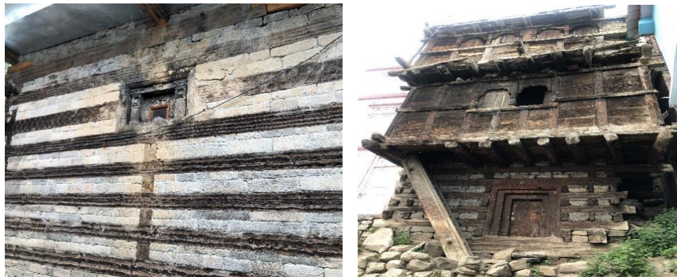
Fig. 1. Traditional Kathkuni Type of Construction in Kinnaur
