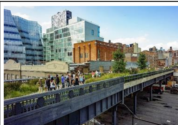
Fig 5. Exterior View of New York High Line Project Source: https://en.wikipedia.org/wiki/High_Line
