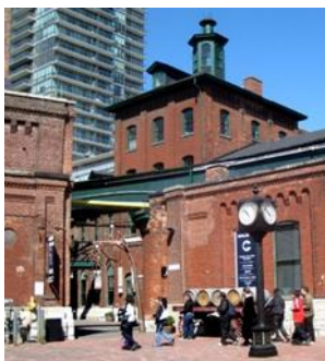
Fig 2. Exterior View of Toronto Distillery District project (TDD)
